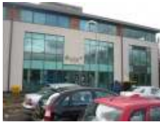
Newbridge Gateway Client: Opco Construction
